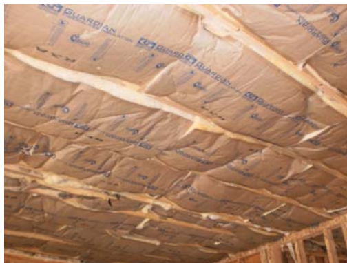
Quality Insulation Installation
