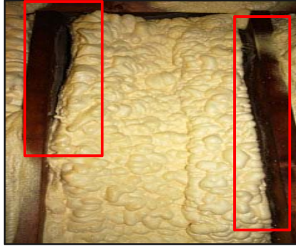
Quality Insulation Installation
