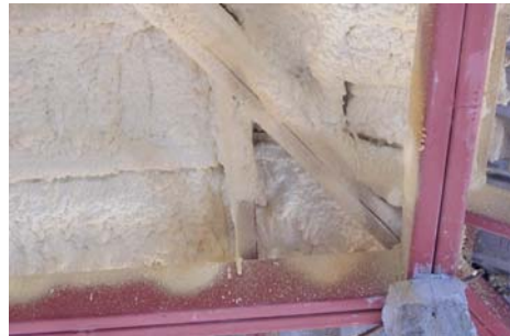
Quality Insulation Installation
