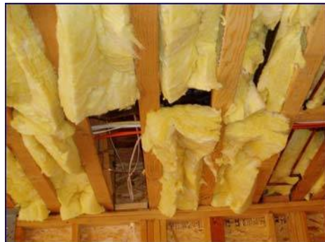
Quality Insulation Installation
