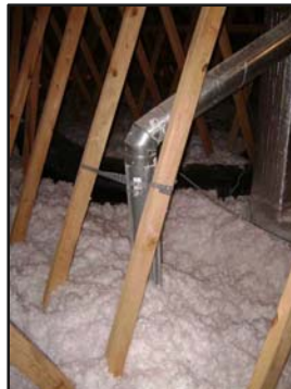
Quality Insulation Installation
