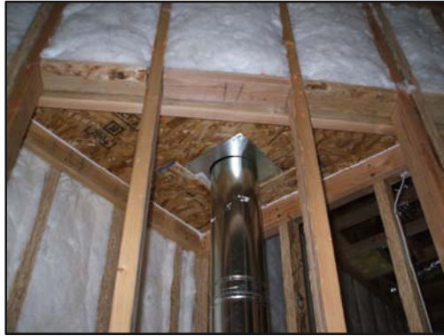
Quality Insulation Installation
