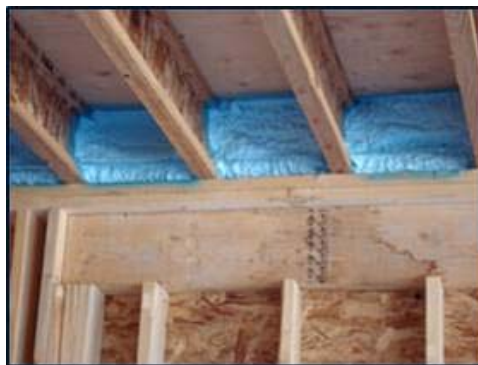
Quality Insulation Installation
