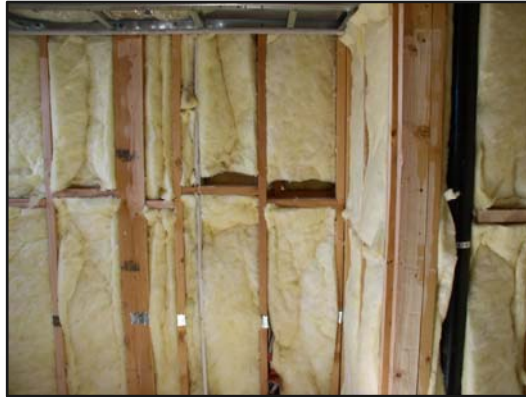
Quality Insulation Installation
