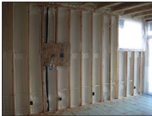
Quality Insulation Installation
