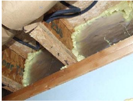
Quality Insulation Installation
