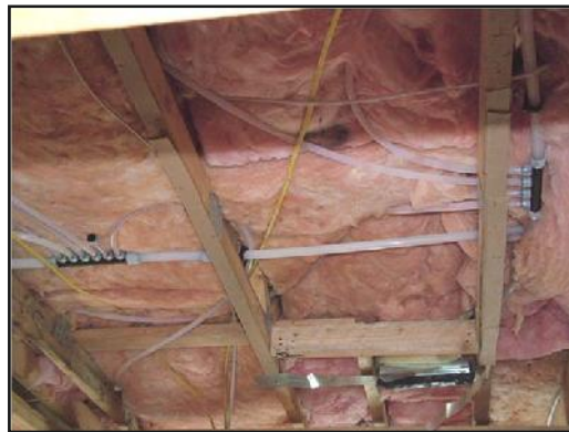
Quality Insulation Installation
