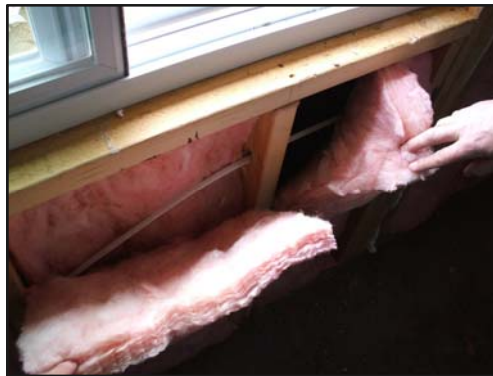
Quality Insulation Installation
