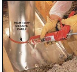
Quality Insulation Installation
