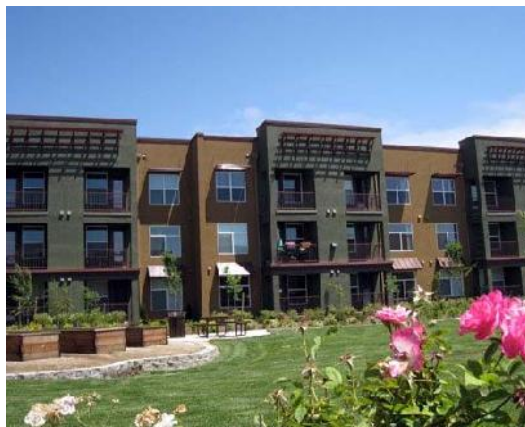
Quality Insulation Installation
