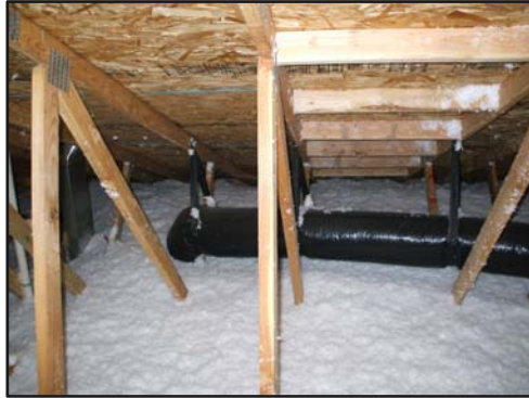
Quality Insulation Installation
