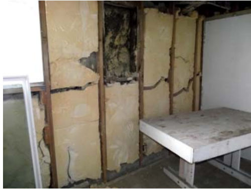
Quality Insulation Installation
