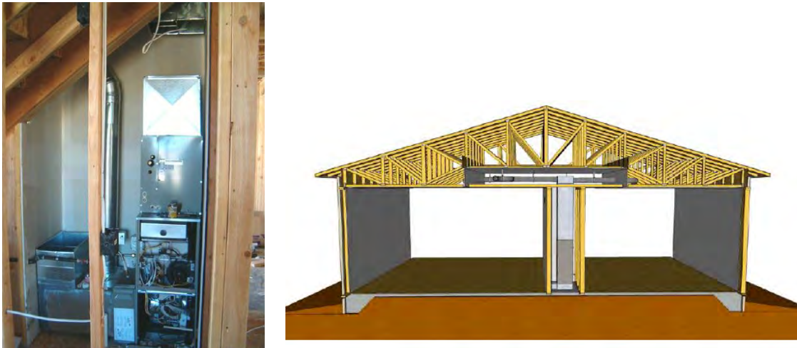
Figure 4-14: Mechanical Closet Placement Example
