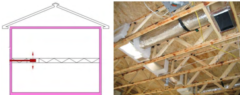
Figure 4-13: Open Web Floor Truss Example
